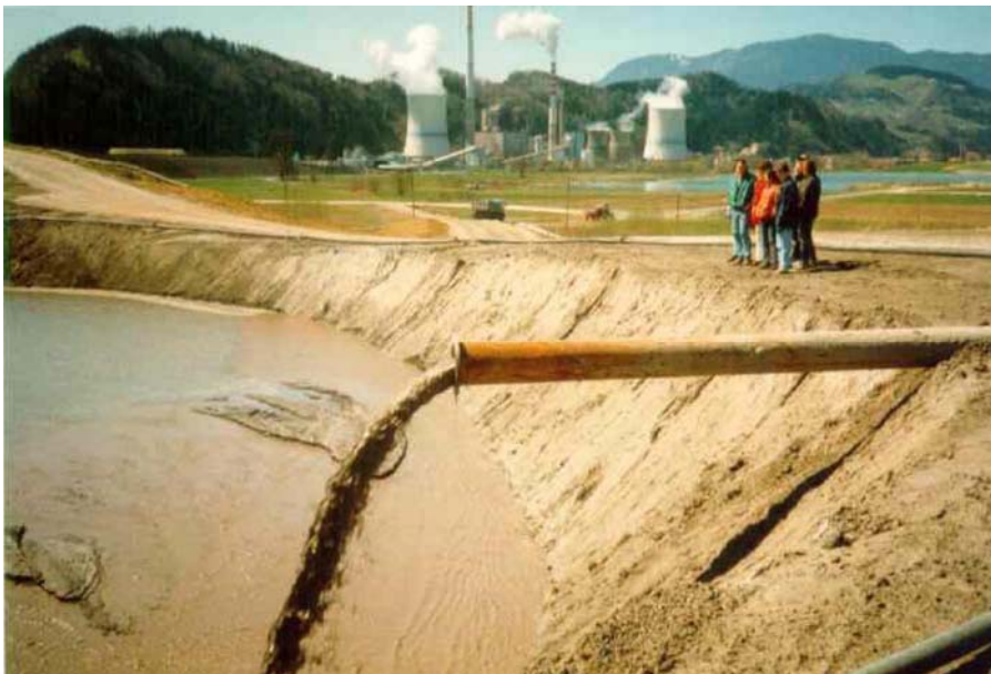
Landfill in Šalek valley
